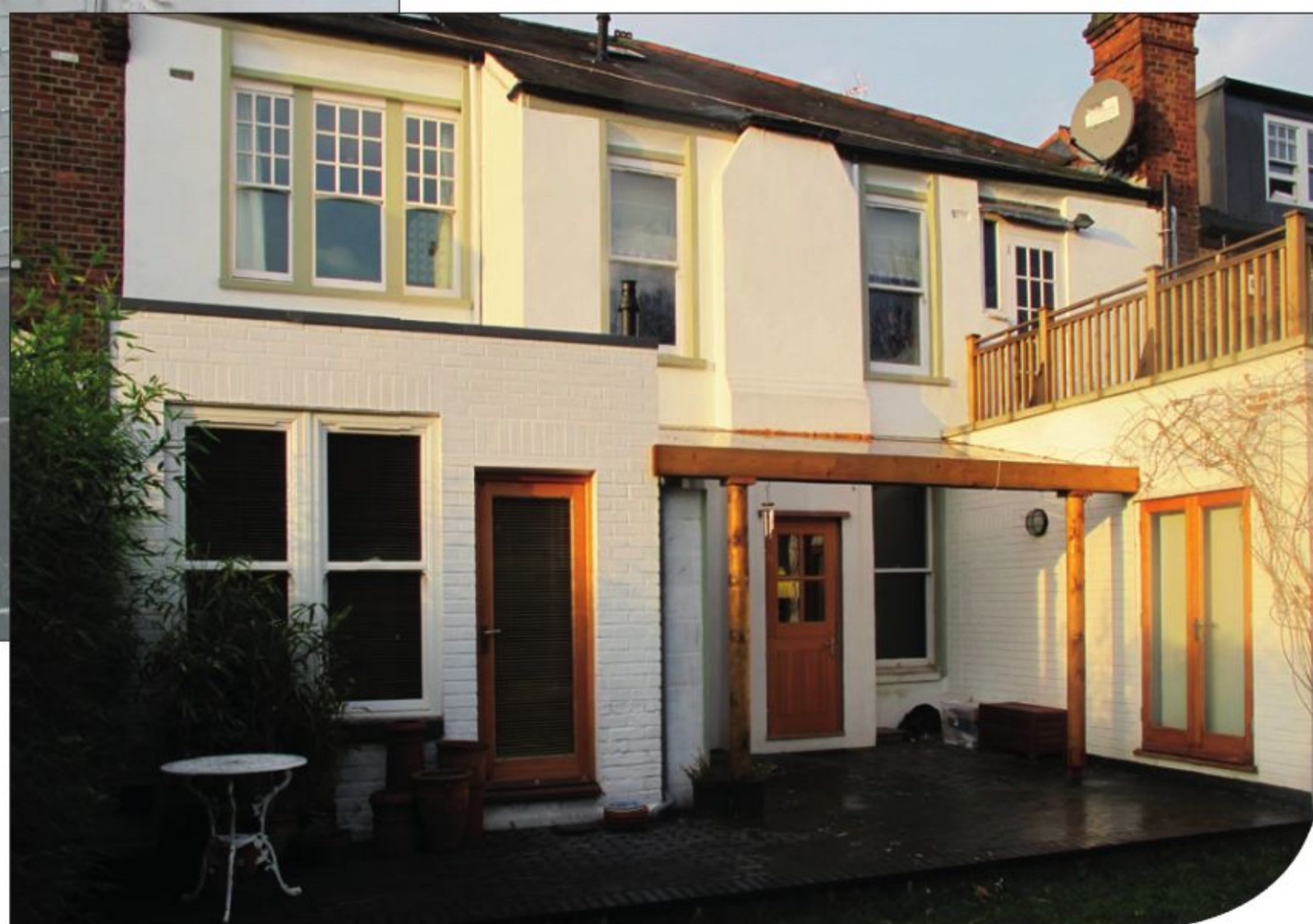
Working space: The boiler was moved to an outside cupboard. For added ease, the Velux windows in Bea's study are operated by remote control
